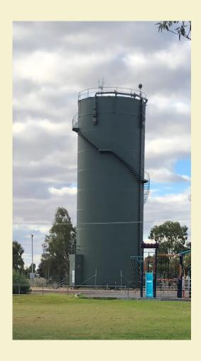
The Whitton Water tower is a metal water tower in use as the town's main water supply. It is painted externally with Marine Grade paint.
